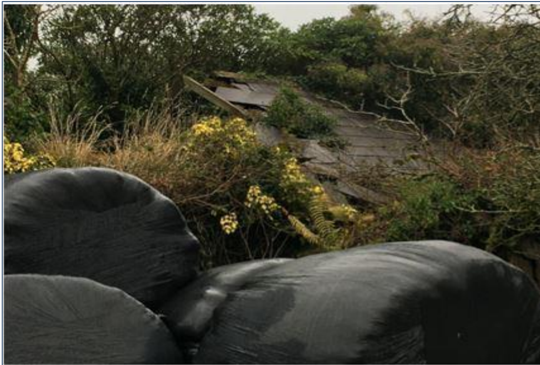
Plate 3-1 Dilapidated Farm Shed
